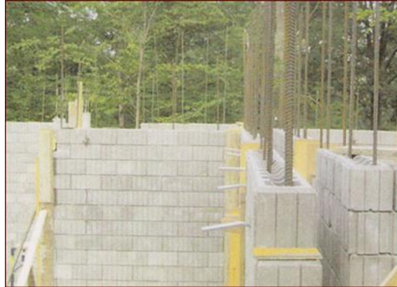
Figure 33: masonry wall construction
