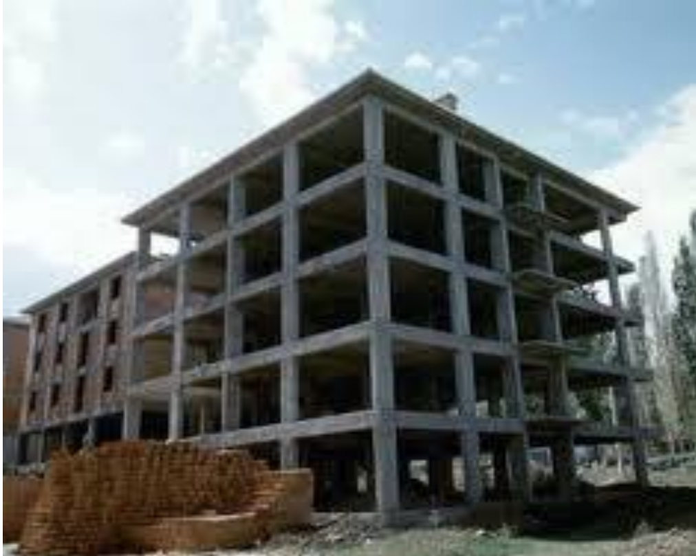
Figure 46: Reinforcement concrete frame
