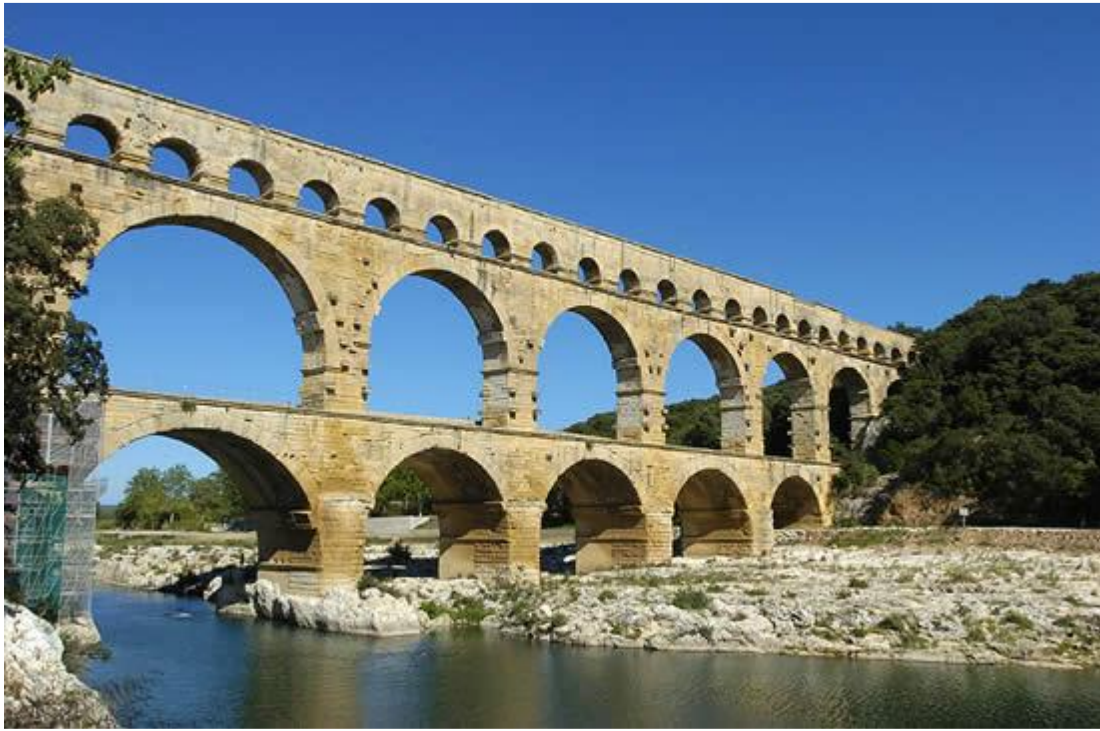
Figure 44: Stone masonry structure
