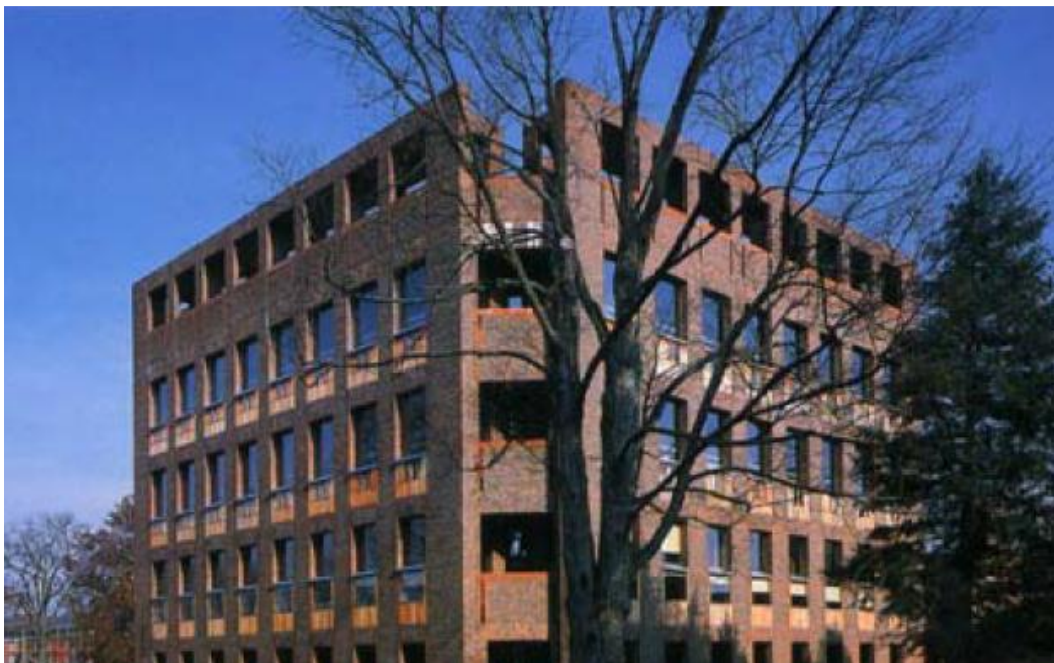
Figure 43: Brick masonry structure
